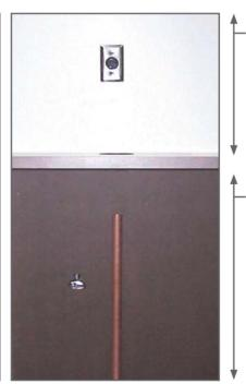
The receptacle, water shut-off valve and drain pipe must be within 3 feet (36"/915mm) of the center of the location (footprint) of the machine.
